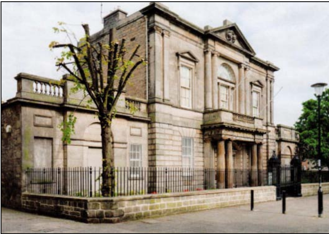
The stately Georgian building incorporates two carved stone panels from the original almshouse.
